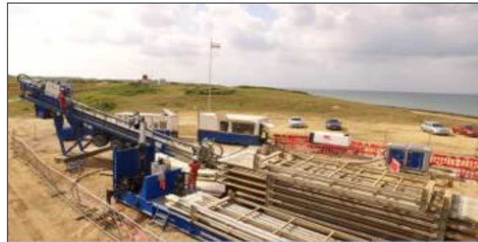
Example Landfall HDD Compound
