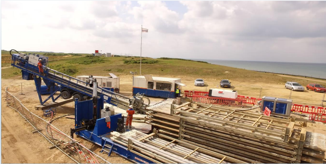
Landfall HDD compound
