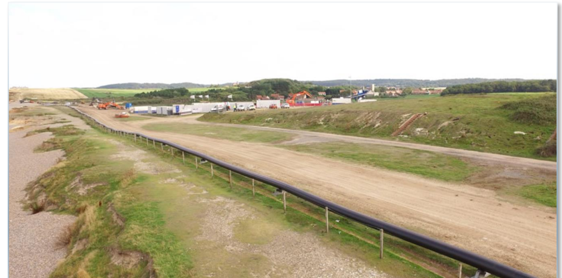
Ducting laid out along cliff edge
