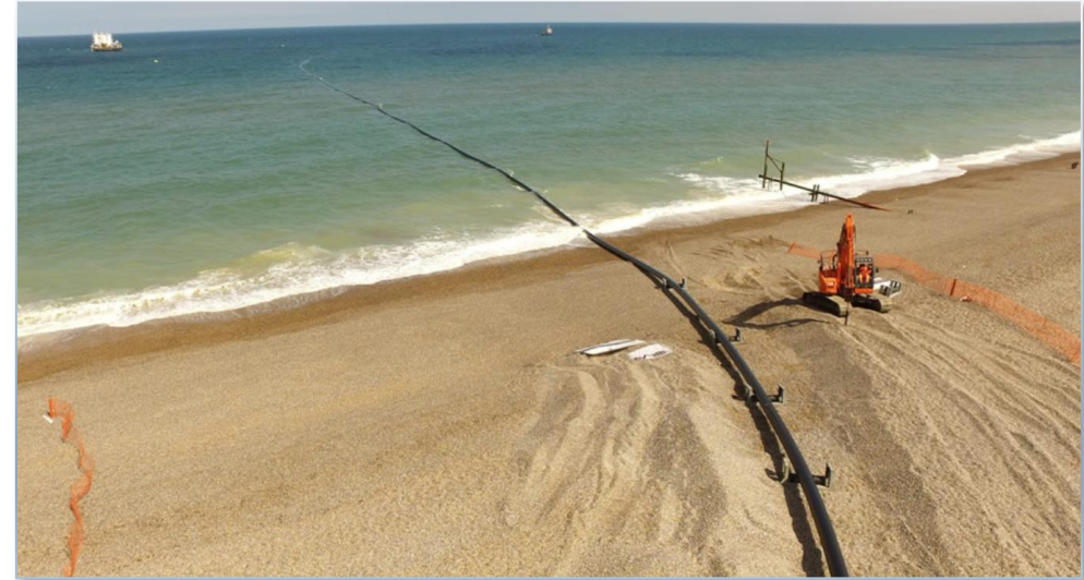
Ducting being towed towards barge
